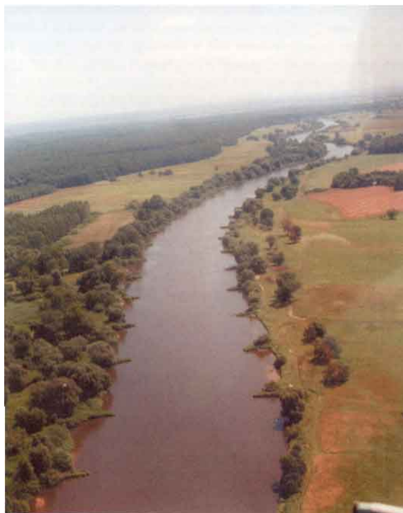
Figure 1.1. Spur-dike on Odra River (IIHR)
